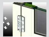
The doors have been designed to accept a heavy adjustable hinge. Screw cover plates removed to show the adjustment screws.
